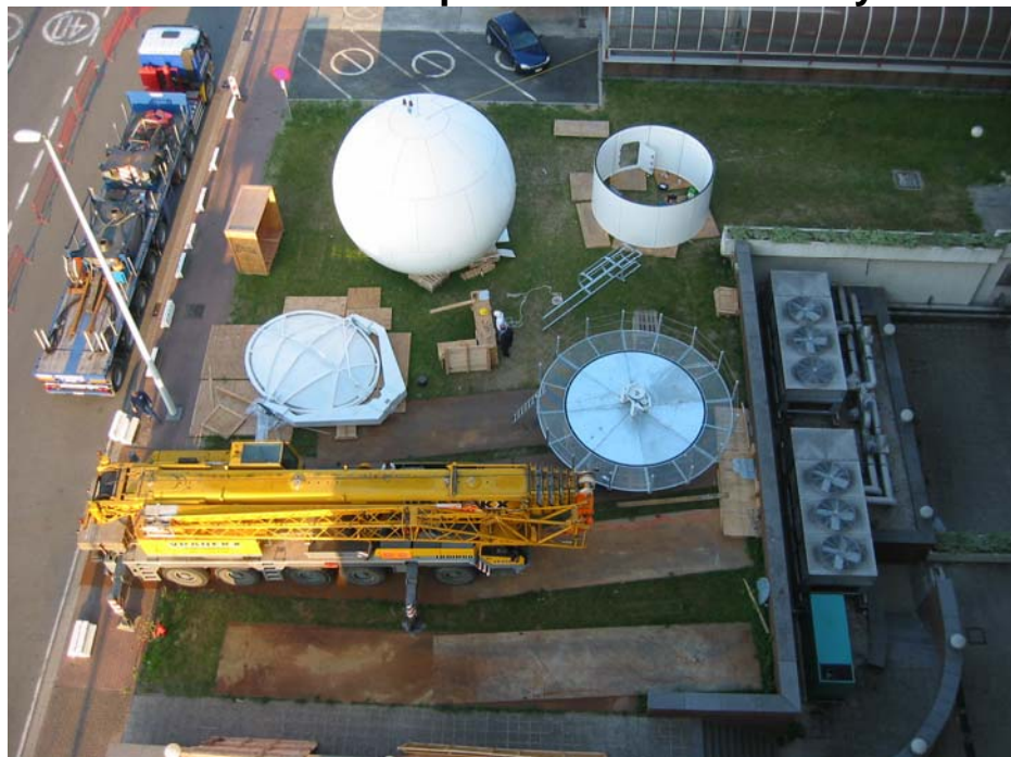
Radome, Antenna and support components prior to lifting into place.
